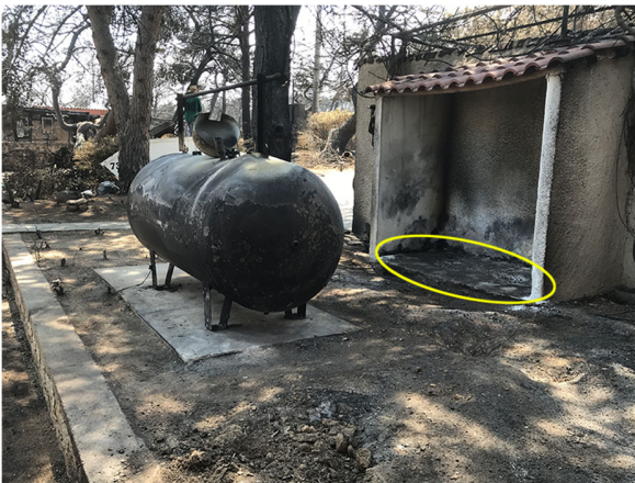
Fig.107. A source of heat may have affected the nearby tank of LPG in Mati (2018).
