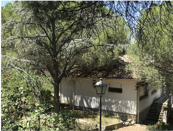
Fig.81. Overhanging tree branches touching the roof of this house in Puentele Sierra, Spain. The accumulation of pine needles is remarkable.
