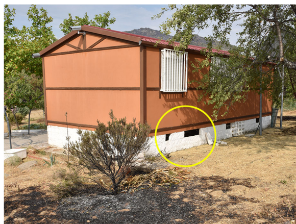
Fig.76. A house with openings in the basement without any protection. Cadalso de los Vidrios, Spain, 2019.
