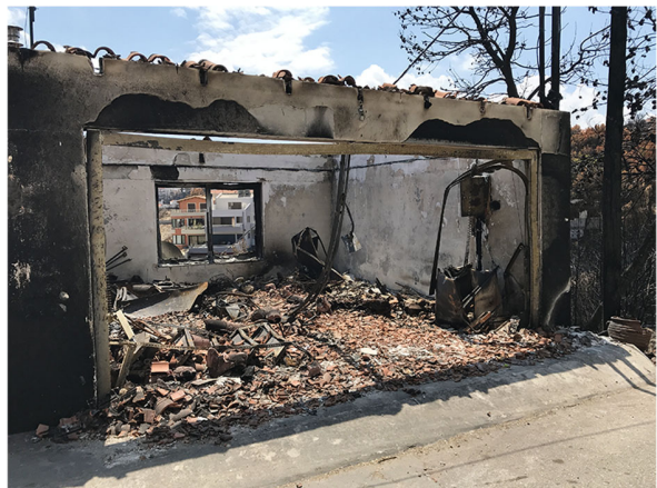
Fig.98.A garage in Neos Voutzas exposed to the passage of the fire and affection to the nearby vegetation, which were touching the structure.
