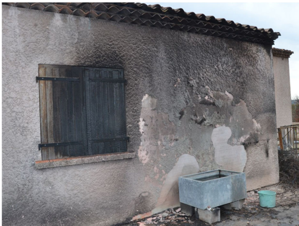
Fig.73. This timber shutter did not sustained combustion in the Rognac fire.
