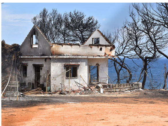
Fig.37. The firefront raged towards the coastline engulfing houses and people. The sea was not a guarantee of survival. Many affected houses have their roofing collapsed. The structure, in many cases, is made of timber.
