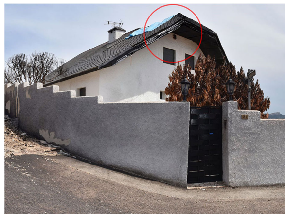
Fig.46. One of the houses receiving direct impact (radiation) over the roofing and affecting the insulation layer in the eave and transferring combustion into the attic.
