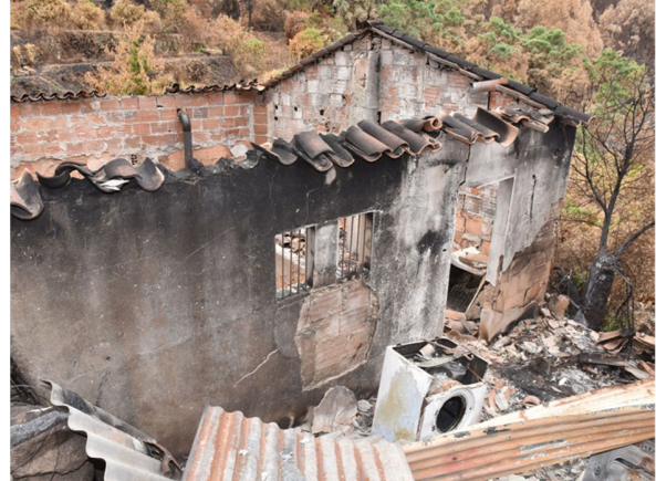
Fig.70. Many of the old houses in Monchique fire (Portugal) had no glazing protecting the windows, hence facilitating the entrance of embers and flames.
