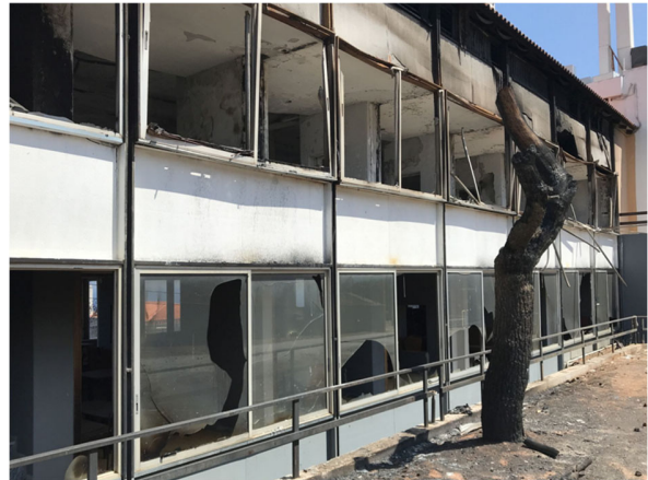
Fig.68. Glazing collapse in Neos Voutzas, as the local effect of the combustion of the touching pine tree.
