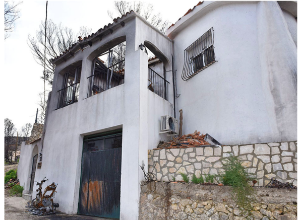
Fig.48. A house severely affected in Montepino settlement. Post-frontal combustion of the many objects and materials in the terrace involved, eventually, the upper part of the building.
