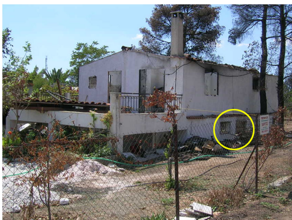
Fig.75. This house shows many entrances to the fire in the basement. Forest fire in Rafina, 2005.
