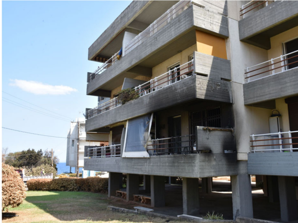
Fig.69. This building in Mati, shows a flat completely burned, as a result of the entrance of flying embers through a window left open.
