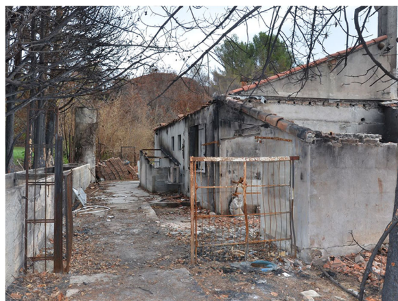
Fig. 21. One of the severely affected houses, with evidence of affection due to firebrands and the combustion of local vegetation near the structure.
