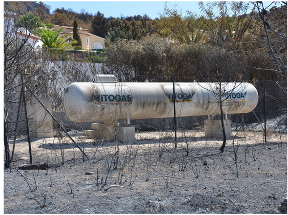
Fig.30. One of the several LPG tanks exposed to the combustion of surrounding vegetation.
