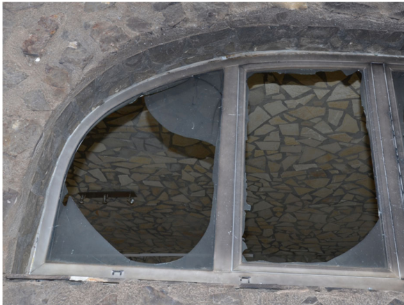
Fig.67. A window pane weakened and finally broken by the effect of the near combustion of a mix of residential and vegetal fuels. Benitatxell 2016.
