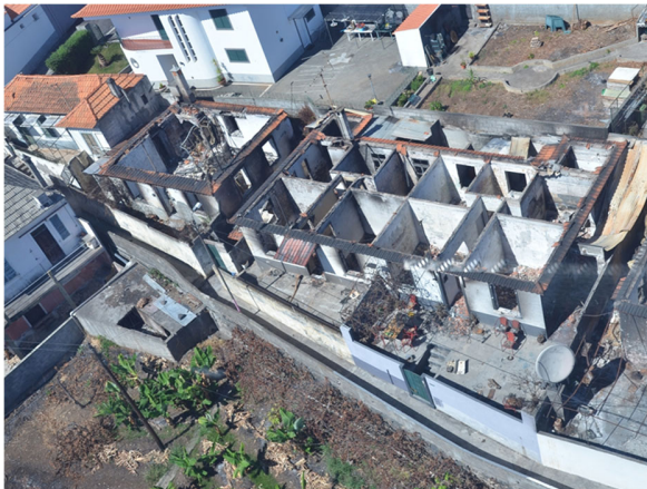
Fig.13. A general view from the cable cabin of the house complex in which three people were killed (lower-right corner). Observe the narrow corridor in the lower part, the only escape to the streets which was compromised as well by the fire.
