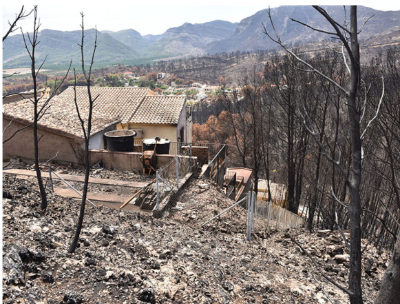
Fig.45. One of the affected houses in the upper part of the settlement of Montepino. The pine stand at the left created a high intensity exposure and projection of firebrands.
