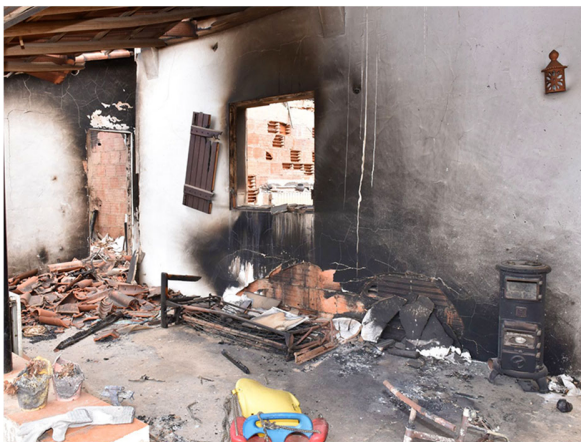
Fig.93. The couch and other materials, ignited by flying embers, are behind the destruction of this house in the Monchique fire, 2018.
