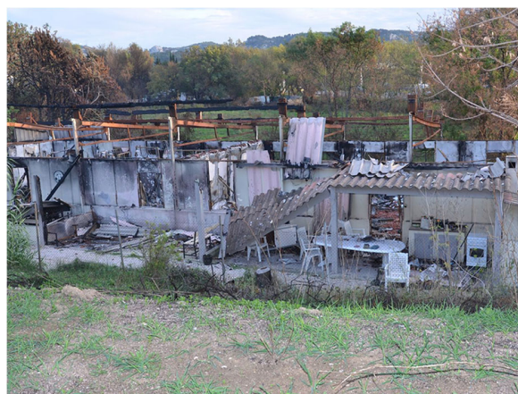
Fig. 23. Given the distance to the main fire front, this structure is likely to be affected by long-distance projected firebrands. Several other houses in the area were unaffected.
