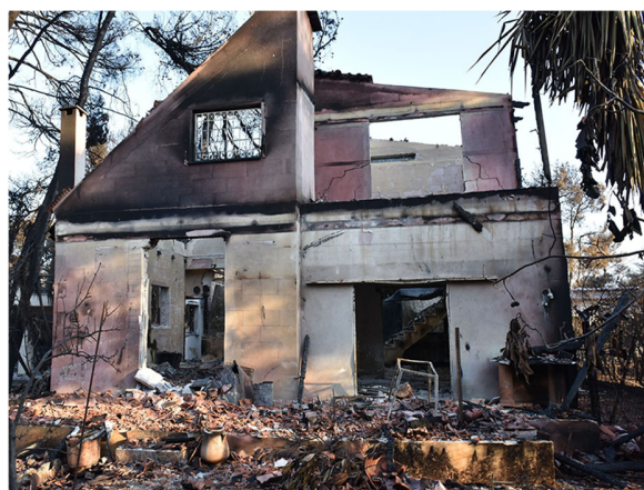
Fig.40. The pos-frontal combustion inside the houses entailed in many occasions the severe affection of the building structure, which was assessed by inspectors in the few days after the event.
