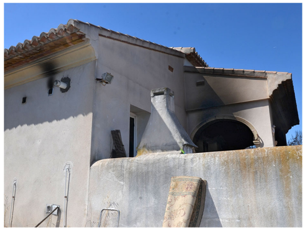
Fig.28. Another house severely affected in the interior. Evidences point to an entrance of firebrands through one of the windows that, presumably, was left open.
