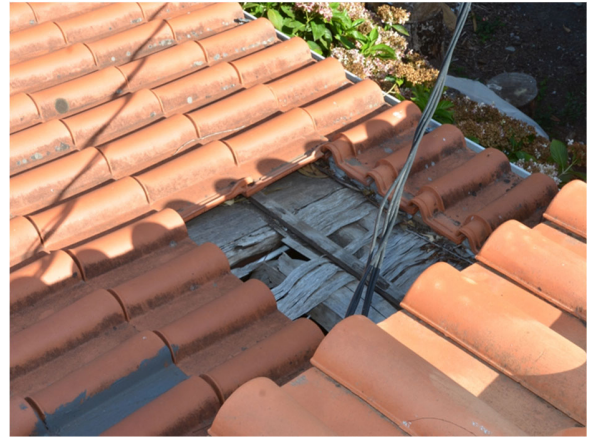
Fig.62. Missing, displaced or broken tiles often expose roofing layering to embers.
