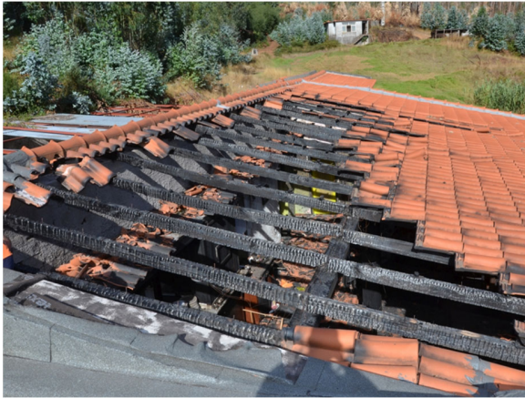
Fig.61. A clay tile roofing affected by spot fires in the Funchal wildfire in 2016.
