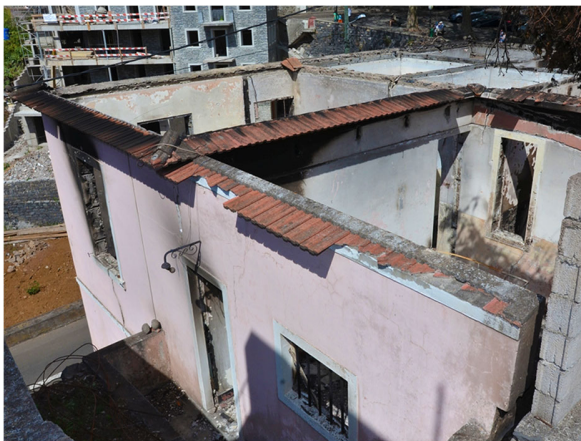
Fig.15. A house completely destroyed with the collapsed roofing in Funchal fire, as a consequence of the fire that propagated from an attached auxiliary building.
