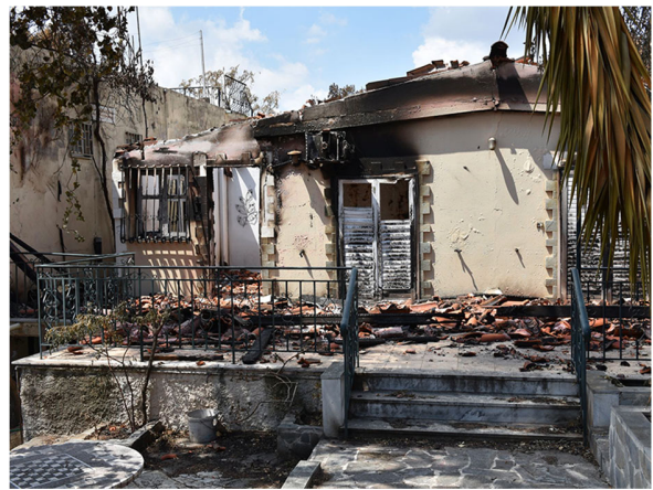
Fig.36. One of the hundreds of structures severely affected or completely destroyed in Mati. Many of the houses showed indication of combustion inside the building.
