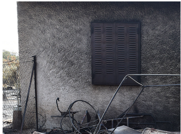
Fig.74. A metal shutter endured the flame impingement due to the combustion of nearby materials and objects in Cadalso de los Vidrios, Spain (2019)
