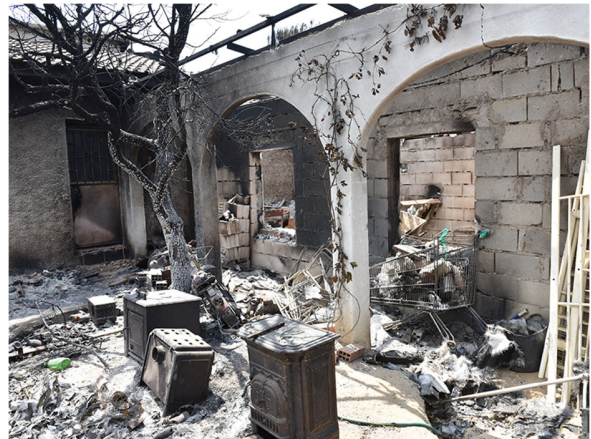
Fig.102. A self-made auxiliary building is completely destroyed due to the combustion of the many objects and materials stored. Cadalso de los Vidrios, Spain, 2019.
