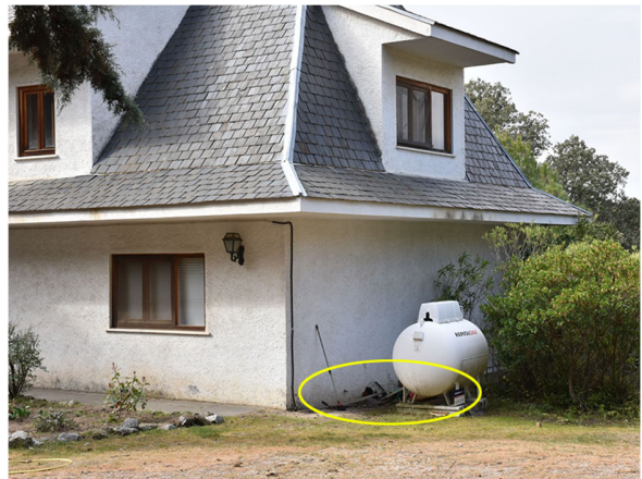
Fig.108. Some objects and materials near this LPG tank and against the wall. In case of a jet fire, a degree of affectation of the house may be expected due to the proximity.
