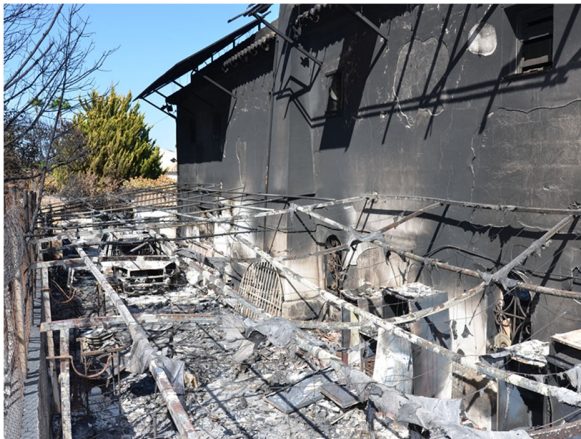
Fig.95.A house severely affected in Benitatzell fire, due primarily to the combustion of the accumulated materials and objects.
