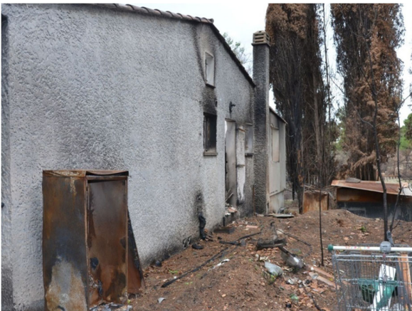
Fig.63. A single point of contact between the cypress and the eave of this house in the Rognac fire entailed the ignition and whole destruction of the building.
