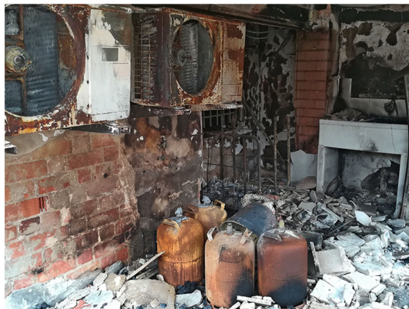
Fig.110. Semi-confined combustion creates a heat accumulation, as the evidence shows in the fire of Lutxent 2018. This lady left the empty canister in the porche, exposing them to sources of heat.
