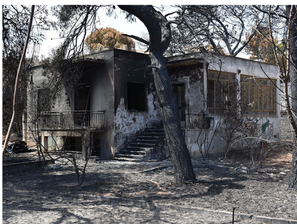
Fig.39. Many of the houses, flat roof, were built in the sixties and seventies, with much less quality on materials and construction standards, which ended in major affections.
