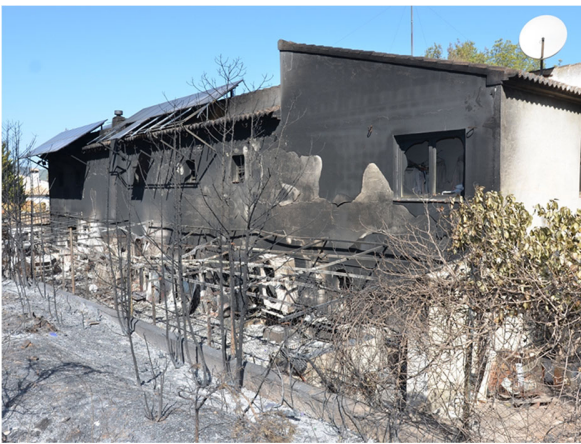
Fig.27. This house received the impact of the left flank of the approaching fire. The existing residential objects and materials entailed the ultimate affection of the house.
