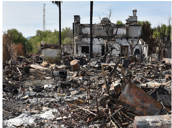
Fig.96.A massive accumulation of objects entailed the destruction of the two houses in the grass fire of Búger, Mallorca (Spain), 2019.
