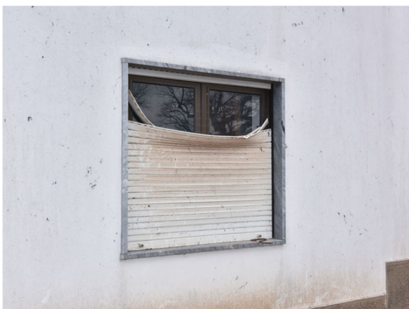
Fig.71. A PVC rolling shutter melted in Monchique fire.
